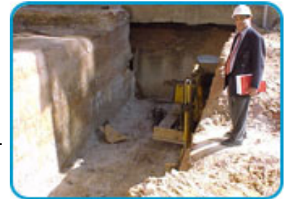
Excavation for Tunnel
